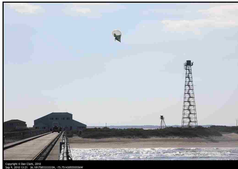
Figure 3.4: Looking onshore from the FRF pier. The FRF imaging tower, located at FRF (x,y) = (33.6\text{m}, 587.1\text{m}) , is 43.3m tall.
